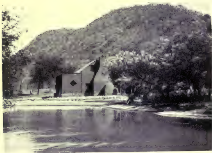
RESERVOIR AT PAVIANSFONTEIN.
